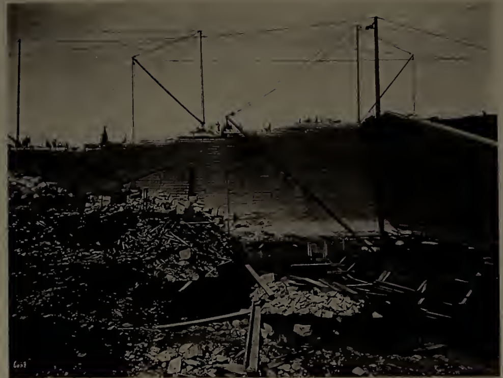
"DAM 5," BOSTON WATER WORKS. Showing work of Contractors Moulton & O'Mahoney.
